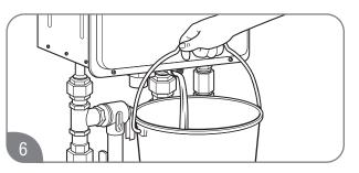
Using a suitable container to catch the water, remove the water filter from the base of the cold water inlet line.
