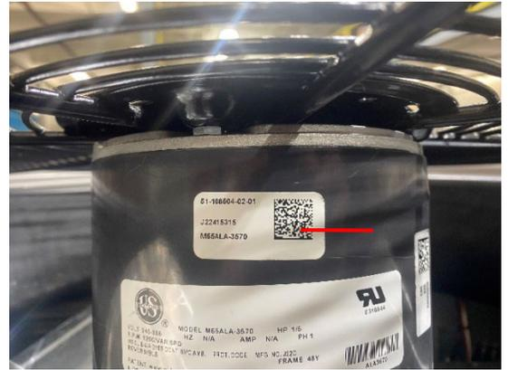
Figure 24. Identify Motor Part Number
