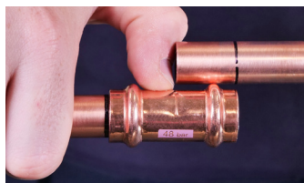
7B. Check the depth mark
