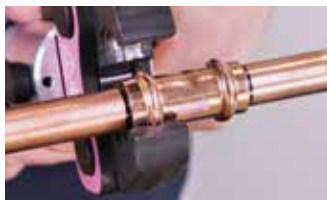
1. Align jaws squarely on the fitting
