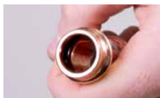
6. Ensure the O-ring is seated
