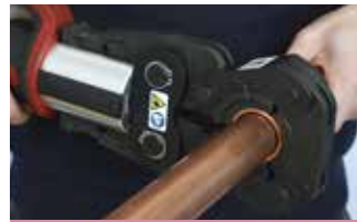
3. Complete the joint with the press tool
