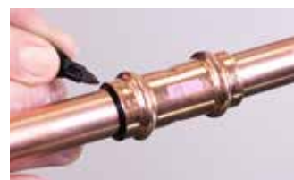
7B. Alternatively insert tube to tube stop and mark
