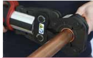
3. Complete the joint with the press tool
