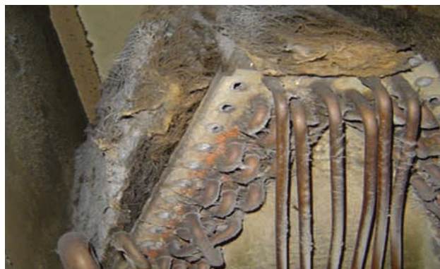
Dirty and frozen indoor AC coil resulting from the use of a standard one inch filter and improper replacement schedule.
